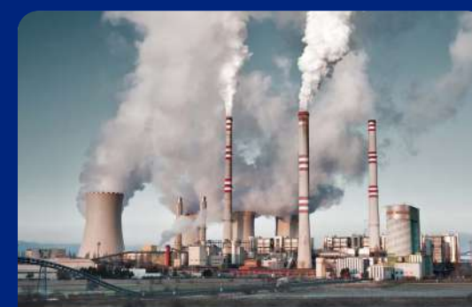
Coal plant decommissioning
